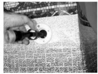
8. Make sure the rubber insert is in place before inserting the lens into the fitting.
