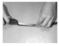
1. Pull the fiber through the wall fitting. With a sharp razor knife, strip off 3-4" of the cable jacket.
