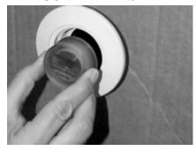
8. Install the lens assembly into the wall fitting. It may be necessary to have someone cautiously pull the cable from the other end.
